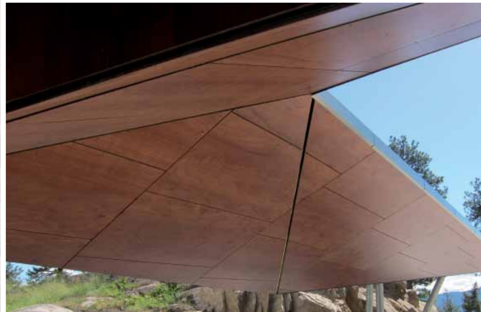
SUSPENDED CEILING: VISIBLE FIXINGS
